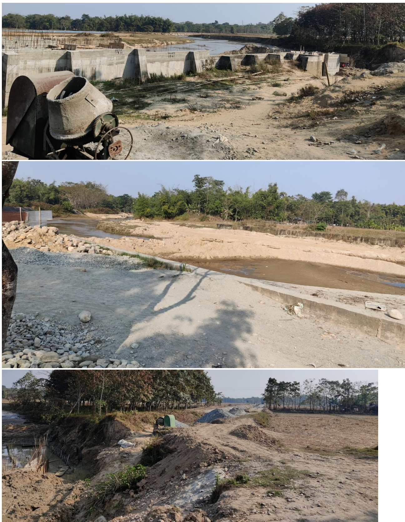
Figure 8: Under-construction Spillway discharging and diverting water from Chandna River to B3M at chainage 16760 m.
